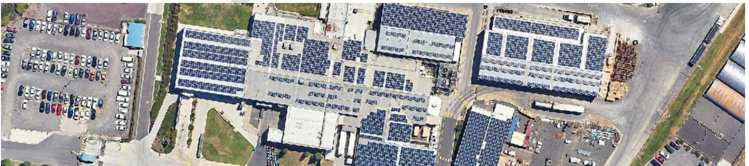
Solar power generation system at the Australian Lamb Company, Colac
