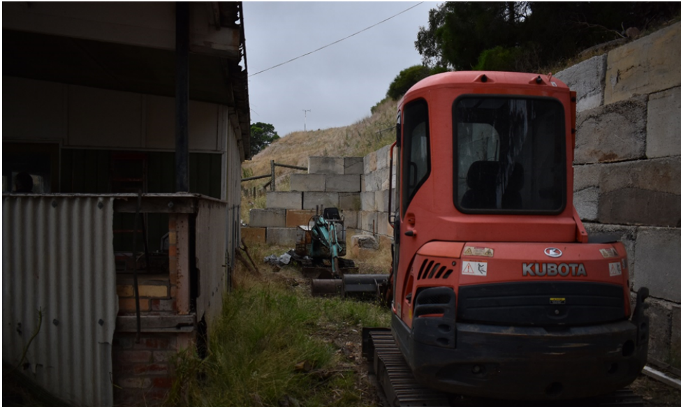
Fig. 17 – Excavator (small) on site
