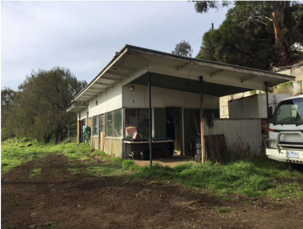
Fig. 13 – Existing building proposed to be converted to a dwelling
