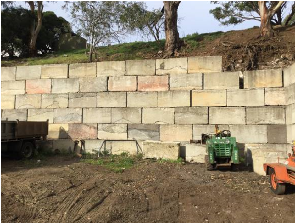
Figure 26 – Existing retaining wall
