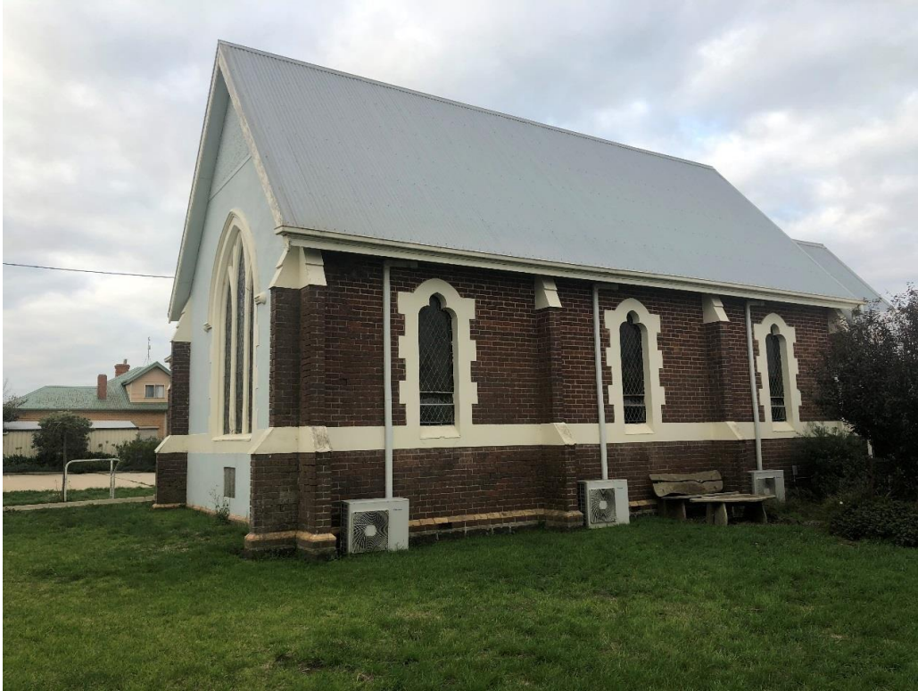
Photo 1: Former St David's Church: south side.
