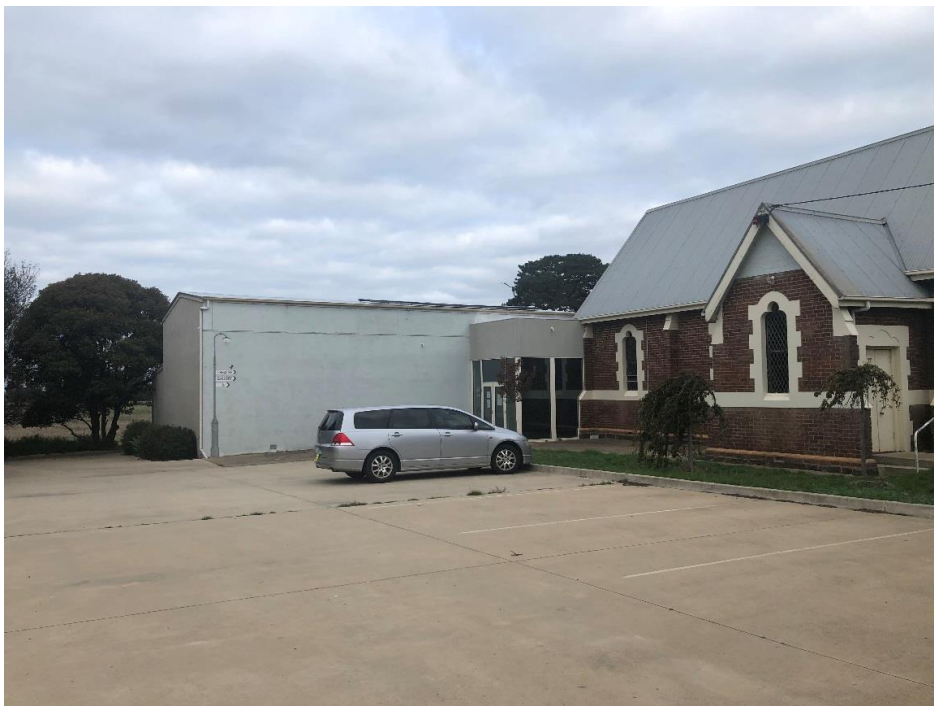
Photo 27: Low fire risk area within the site.
