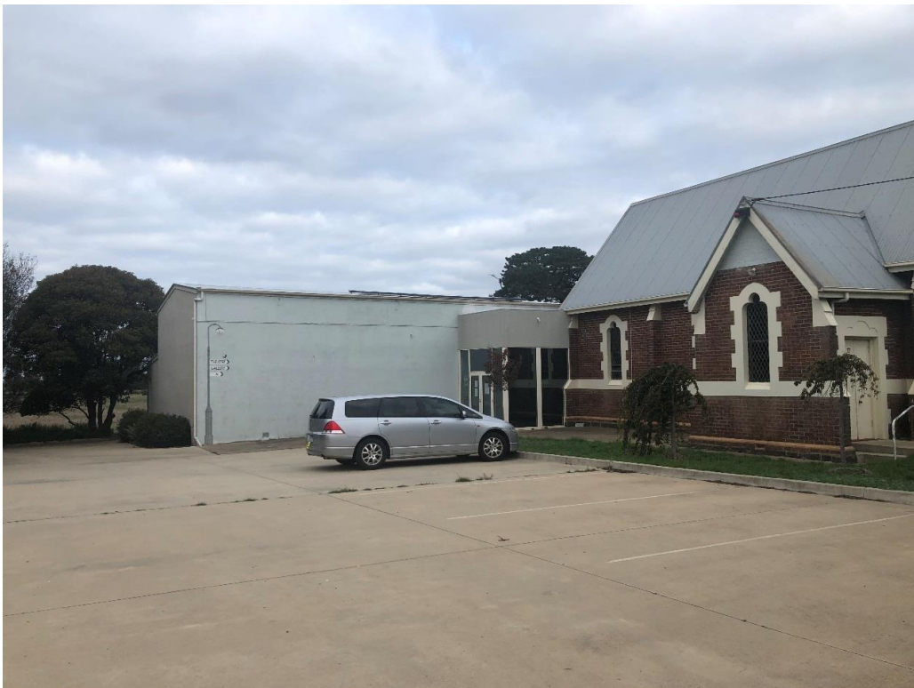
Photo 12: Existing car park & entry.
