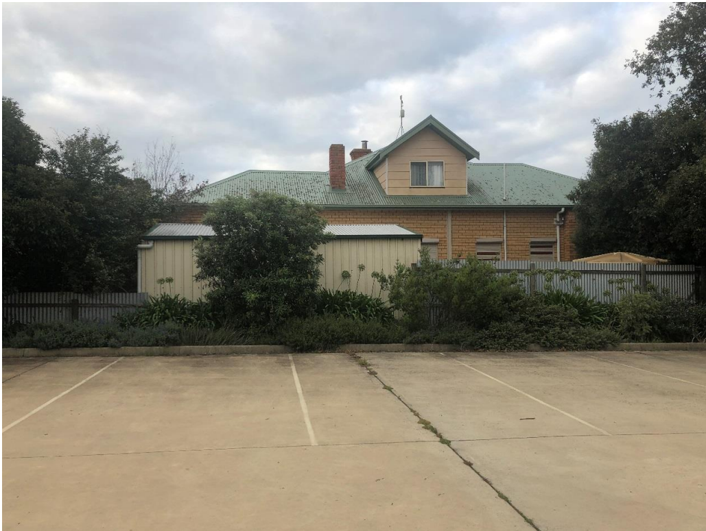
Photo 34: View to north. Dwelling as exclusion.
