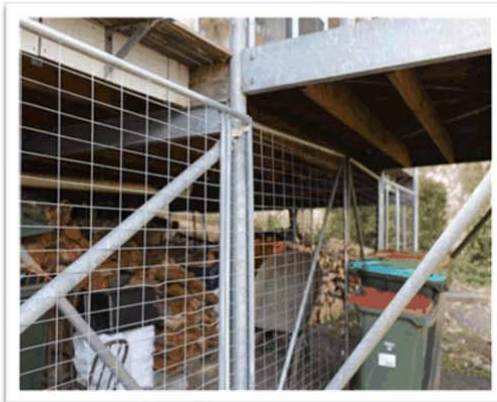
Figure 31 Heavy fuel stored under a house
