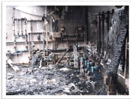
Figure 32 and Figure 33 Damage to a water pumping plant which occurred during the 2009 Black Saturday fires
