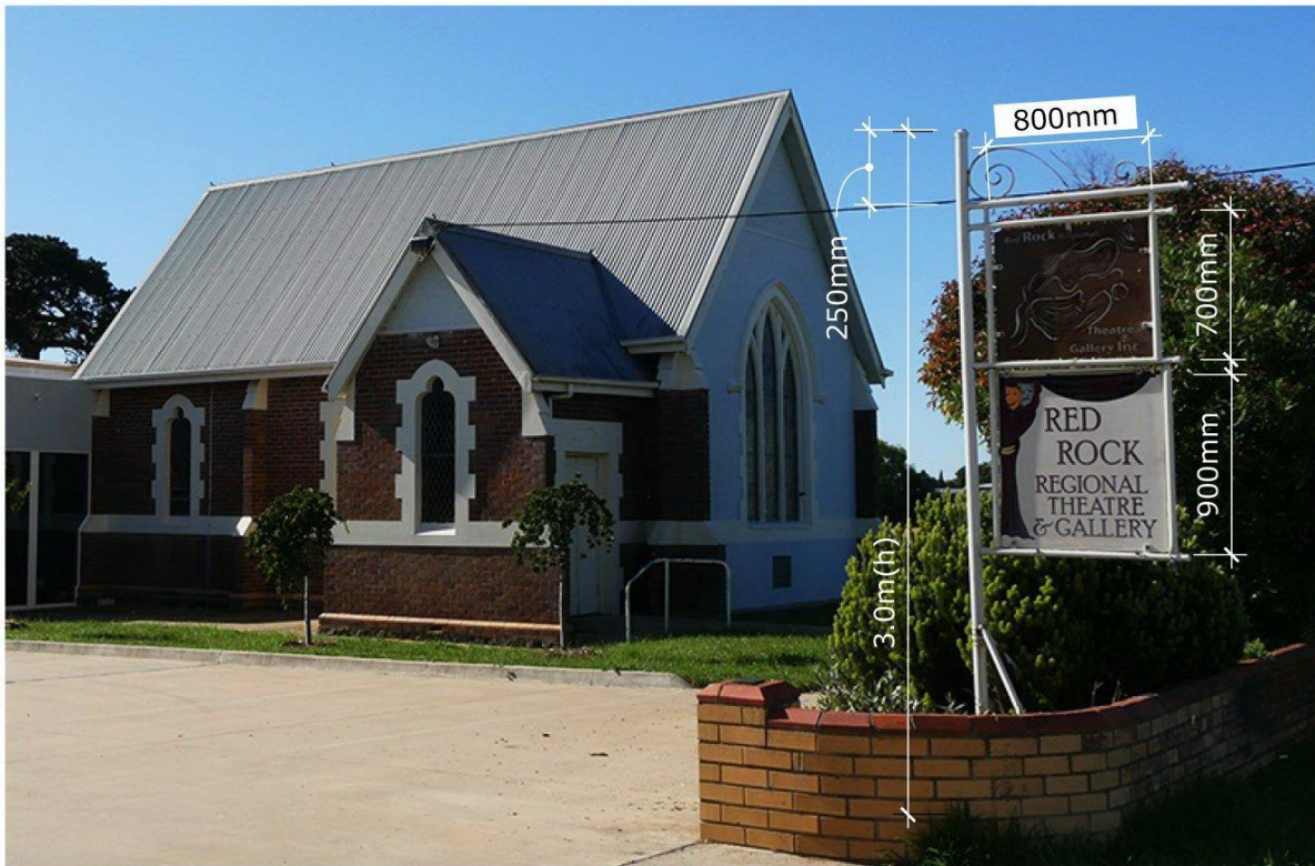
Existing signage (above). 'Now Open' sign (as shown below) is currently utilised and hung from frame with hooks and eyes.
