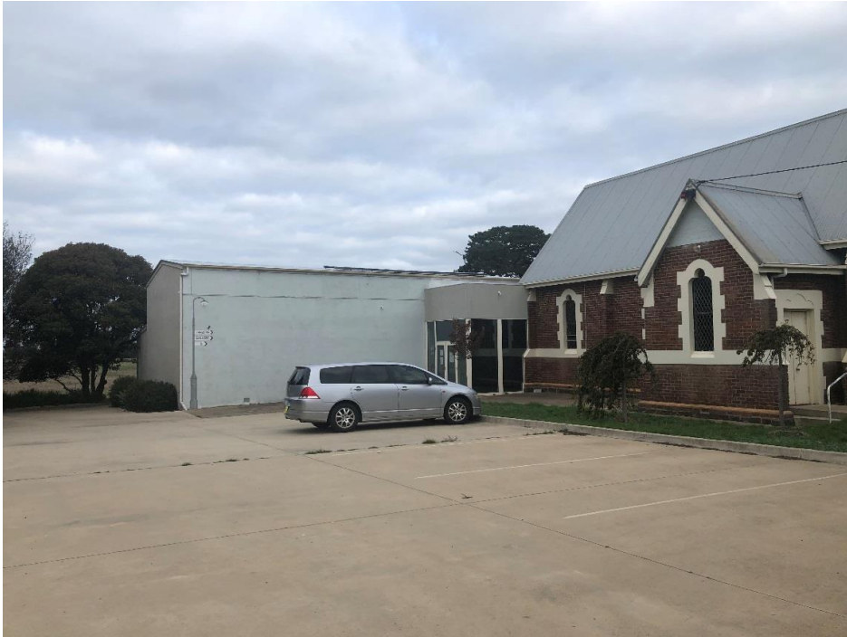
Photo 27: Low fire risk area within the site.
