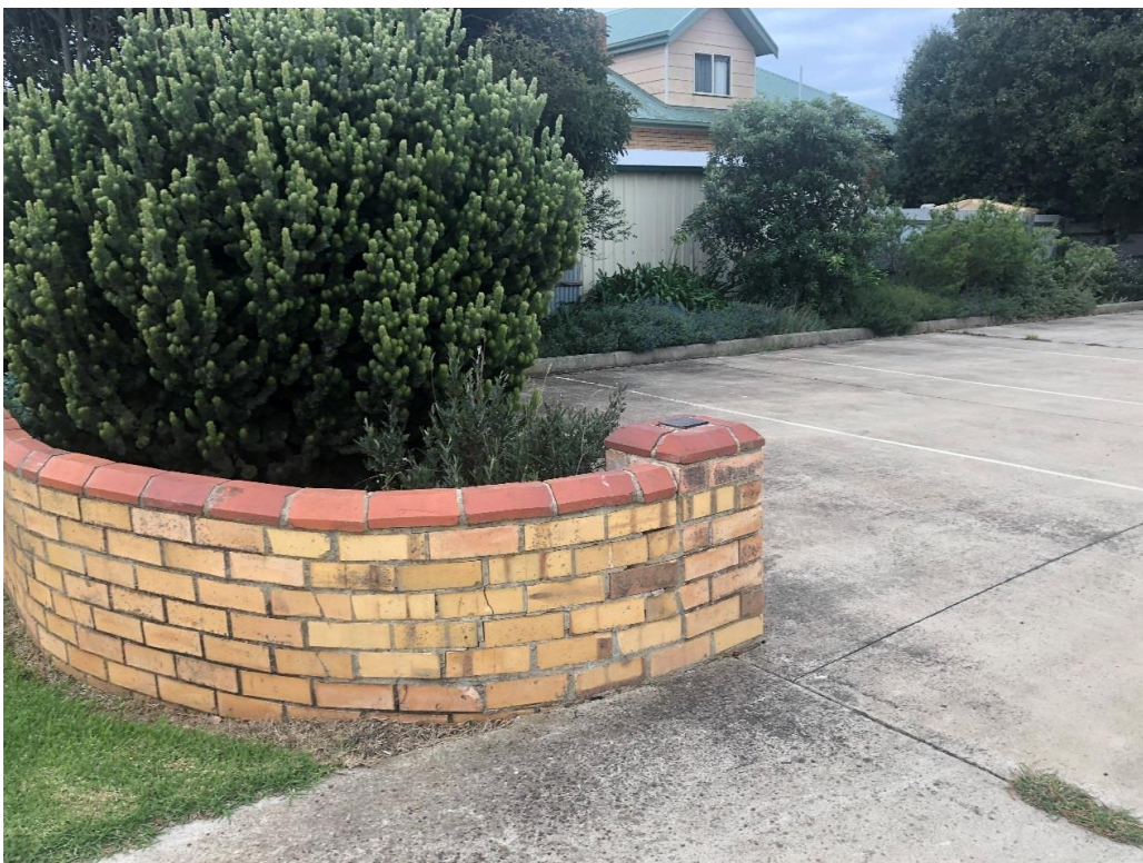
Photo 10: Existing entry and fencing.
