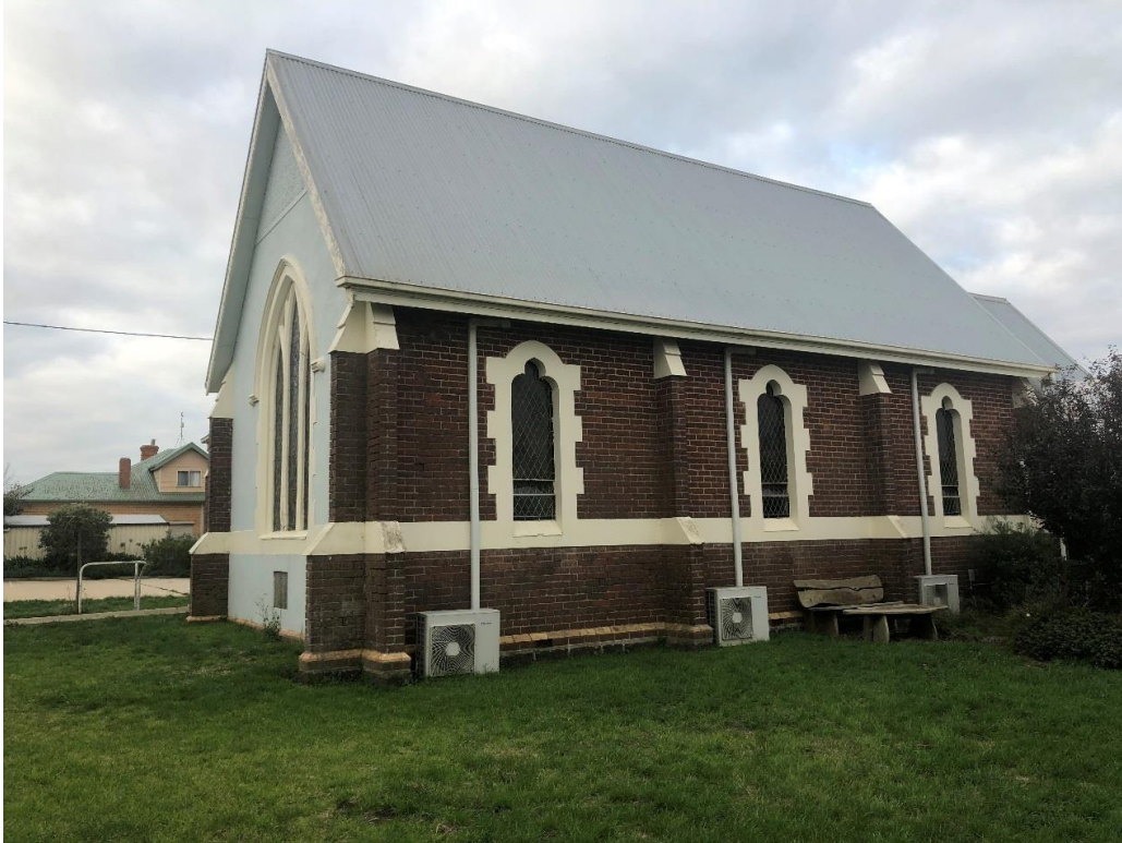
Photo 1: Former St David's Church: south side.
