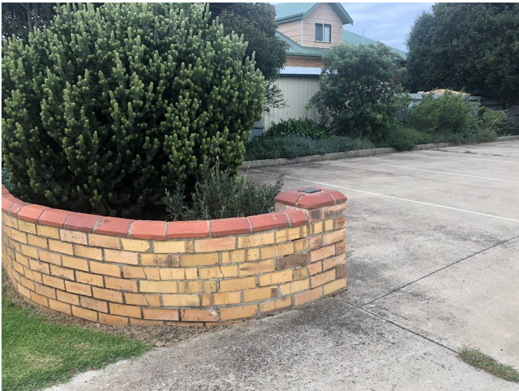
Photo 10: Existing entry and fencing.
