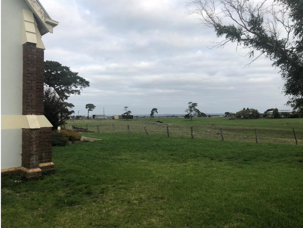
Photo 13: South side of former church
