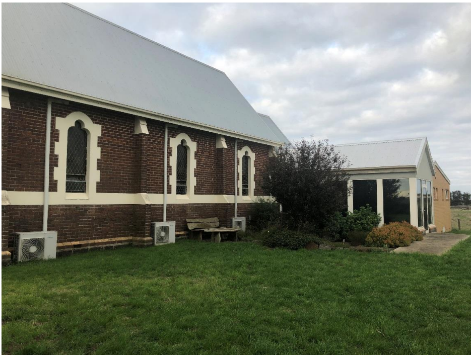
Photo 28: Southern façade existing gallery and hall buildings.
