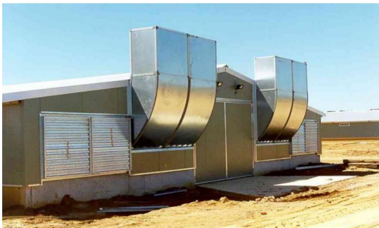
Figure 8-1 Example of stub-stack tunnel ventilation
