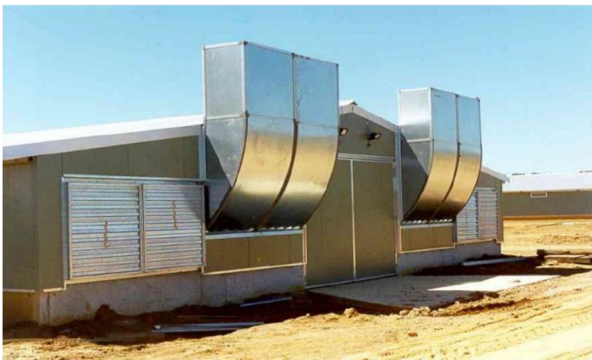
Figure 8-1 Example of stub-stack tunnel ventilation
